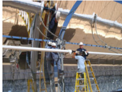
Hands-on approach in support of power from the desert. Assembly of reflectors for a demo-version of a parabolic trough system, assembly of absorber pipes. Source: Solar Millennium AG
