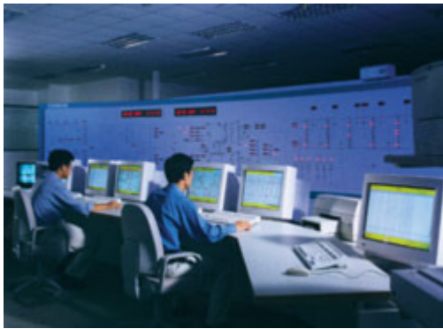
Left: Control room of one of the two frequency converting stations of the HVDC transmission line (1 800 MW) covering 960 km between Tianshengqiao and Guangzhou in China. Right: Thyristor ventilators of an HVDC line in China. Source: Siemens AG.
