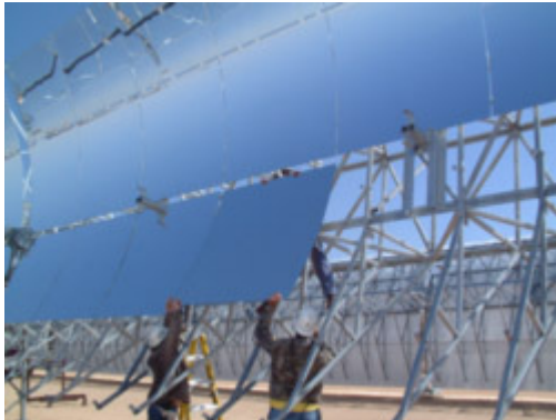
Hands-on approach in support of power from the desert. Assembly of reflectors for a demo-version of a parabolic trough system, assembly of absorber pipes. Source: Solar Millennium AG
