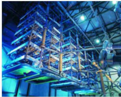
Left: Control room of one of the two frequency converting stations of the HVDC transmission line (1 800 MW) covering 960 km between Tianshengqiao and Guangzhou in China. Right: Thyristor ventilators of an HVDC line in China. Source: Siemens AG.
