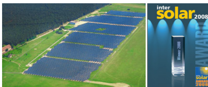
Solar park "Rote Jahne I" (6 MWp) is monitored by skytron surveillance solutions. Photo: Juwi Solar GmbH
