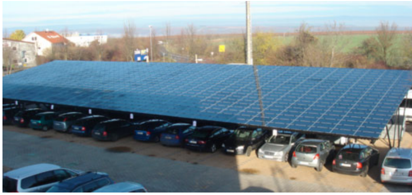
Solar carports will be the fueling station of tomorrow.
