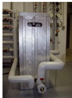
Left: Buffer storage unit of the solar system in the student village of Freiburg Vauban. Right: External heat exchanger. Photos: Hochschule Offenburg.
