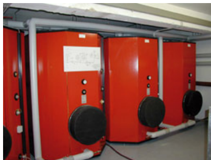
Left: Buffer storage unit of the solar system in the student village of Freiburg Vauban. Right: External heat exchanger. Photos: Hochschule Offenburg.
