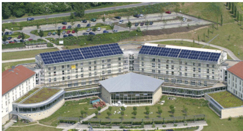
Solar heating system in the Rehabilitation Clinic Bad Frankenhausen. Source: Xtoday-Media Verlag; TU Ilmenau
