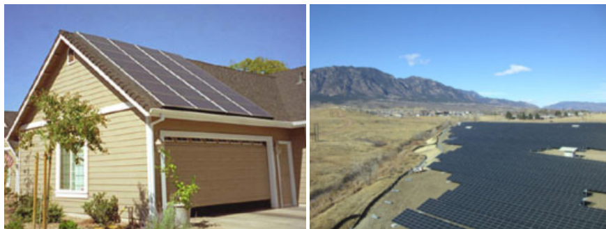
PV generator(3 kWp ) on the roof of a garage in California; aerial photo of the 2 MW solar power plant at Fort Carson. Sources: Evergreen Solar, Inc.; Conergy AG
