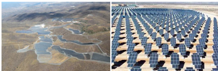
Left: 23 MW solar energy system in Spain; right: 15 MW solar PV installation at Nellis Air Force Base (Nevada). Sources: Munich Energy Partners; U.S. Air Force
