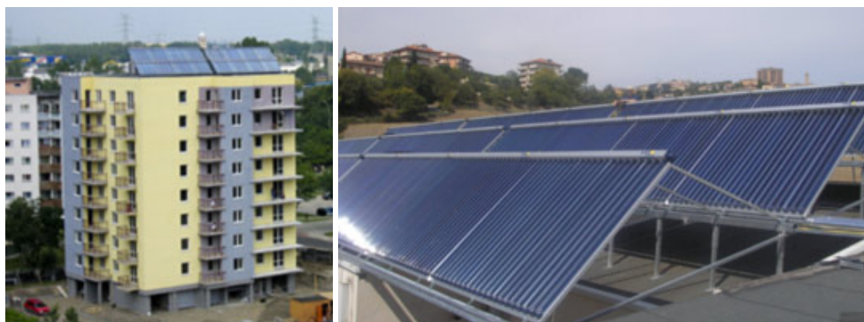
Left: Large-scale solar thermal system of a multi-storey apartment building near Katowice (Poland). Right: CPC collectors of an indoor and outdoor swimming pool in Ancona (Italy). Photos: Paradigma Energie- und Umwelttechnik GmbH & Co. KG.
