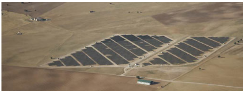
3,26 megawatt solar power plant in Albacete, Spain.
