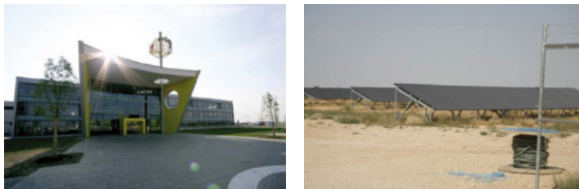
CISfab of Würth Solar; Detailed view of the plant in Albacete.
