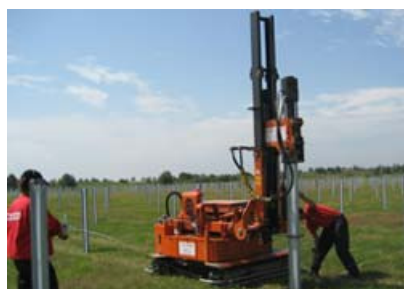
Left: 30,000 posts had been rammed into the ground. Right: solar module frames made of aluminum.
