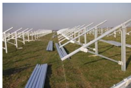
Left: 30,000 posts had been rammed into the ground. Right: solar module frames made of aluminum.
