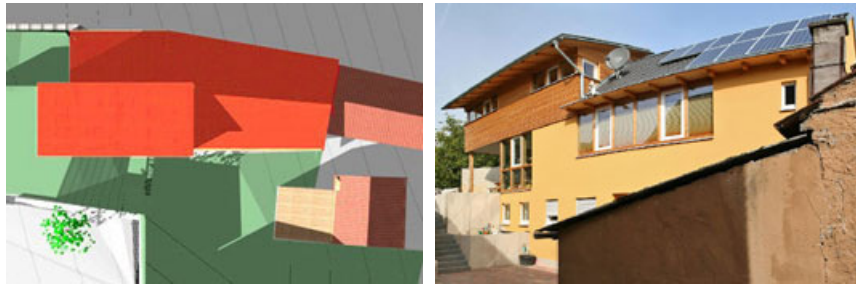
Left: With a CAD model the shading study was carried out in order to optimally utilise solar energy passively (direction of windows) as well as actively (orientation of solar modules); right: partial view of the solar generator.
