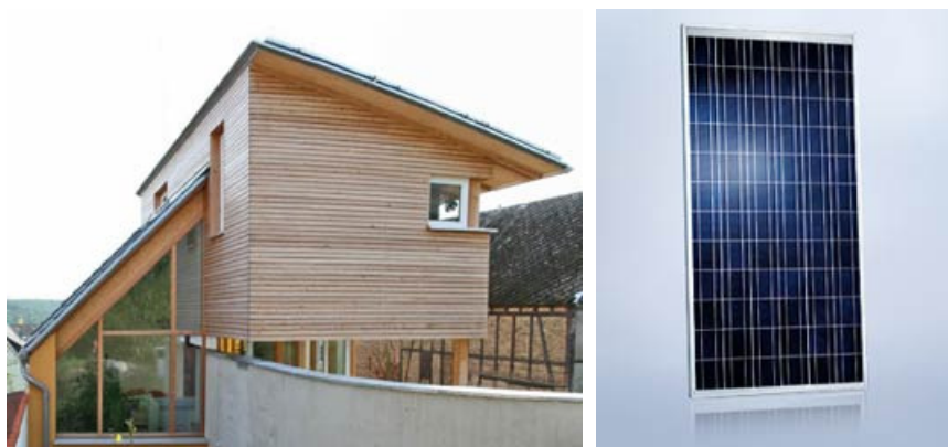
View from the garden onto the building: on the main roof with a pitch of 19°, 36 solar modules from SCHOTT Solar have been mounted. Sources: C. Dahl; SCHOTT Solar AG.
