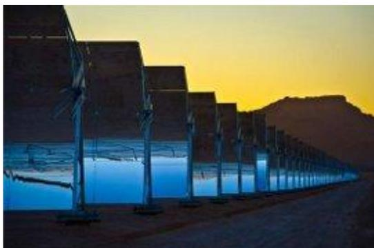
*The Solana CSP plant can produce six hours of electricity without operation of the solar field*
