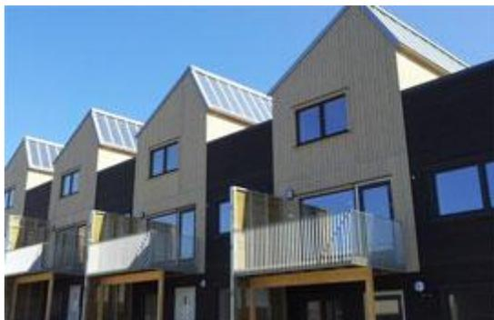
Sixty-two per cent of the total energy consumption for both space heating and hot water are supplied by the polymeric solar collectors. The model housing estate for energy-efficient building became a benchmark project for the solar and building sectors, fulfilling the aspirations of both architects and building owners. [More](#)
