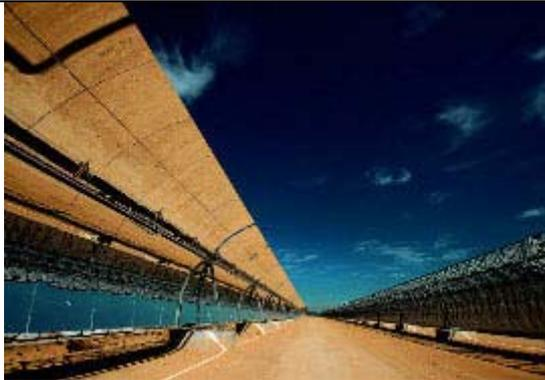
The Indian plant utilizes parabolic trough technology
