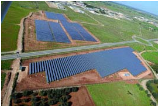
PV plant in Apulia, Italy. Picture courtesy: SunEdison
