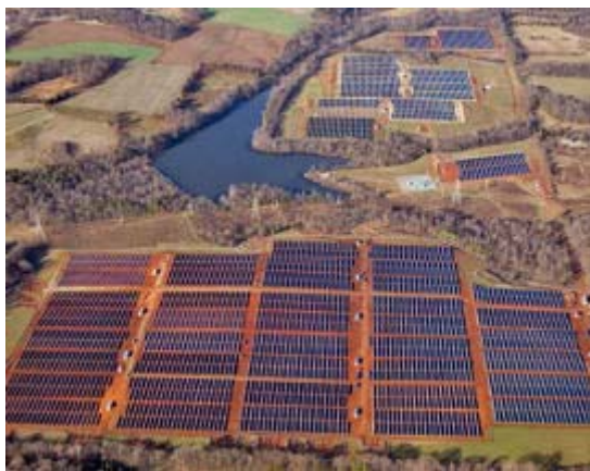
Sun Edison/Duke Energy PV plant in Davidson County, North Carolina
