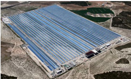
Also in Spain, late last week Novatec Solar commissioned the 30 MW Puerto Errado 2 CSP plant, as the world's largest linear Fresnel CSP plant. PE2's solar boiler includes a mirror surface of 302,000 qm making it the world's largest operational solar thermal power station based on linear Fresnel collector technology. [More](#)
